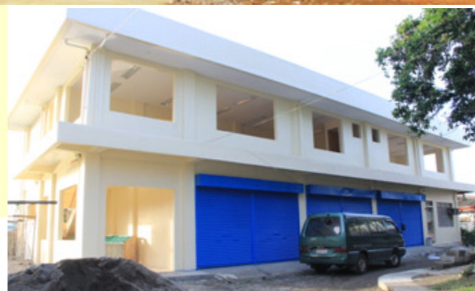
Completion of Stock room/maintenance building
