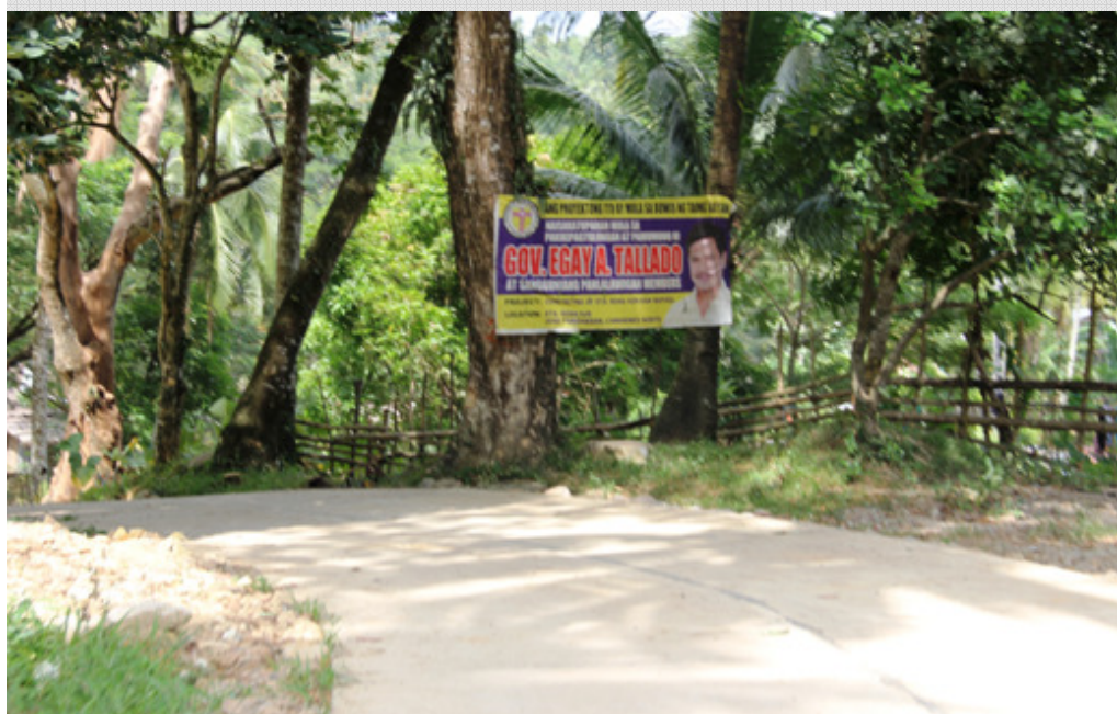
JOSE PANGANIBAN —Sta. Rosa Sur-San Rafael 2.81 Km Farm to Market Road, with P20 Million funding from OPAPP-PAMANA thru the intercession of HON. GOV. EDGARDO A. TALLADO
